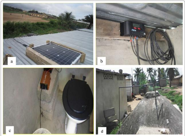
Fig. 2 A single-stage solar-supported hyper-thermophilic anaerobic biogas digester constructed in Terterkessim slum, Elmina (Source: [21]). a Solar photovoltaic, b charge controller, c a pure sine wave invertor kept near the toilet seat, d single-stage solar-supported biogas digester
