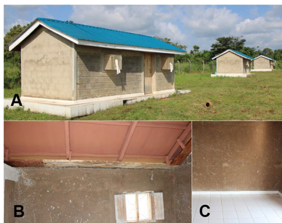
Fig. 1 Experimental hut design: A front view of the hut fitted with window exit traps, B showing the wood baffles, and C showing the tiled floor and the hut interior walls
