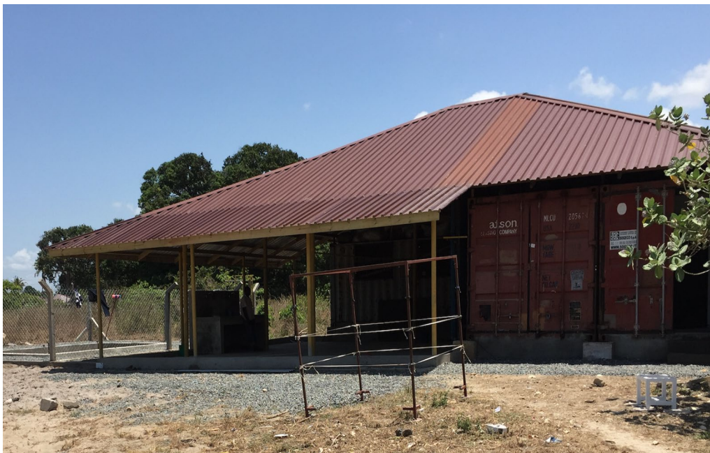
Fig. 1 The Bagamoyo IHI LLIN storage facility
