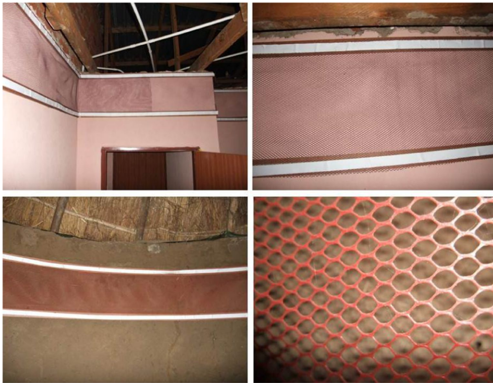
Fig. 2 ITWL installed in community dwellings. A purple (0.85 wt% deltamethrin) lining attached with Velcro® to a wooden frame mounted against the interior wall of a bedroom in a study house ( top left ). The section of overlap for efficacy sample testing is above the doorway. A close-up of the lining and attachment method ( top right ). An orange (0.47 wt% alpha-cypermethrin) lining installed in a sleeping hut ( bottom left ). A close-up of the extruded mesh ( bottom right )
