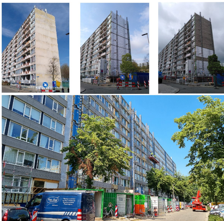
Fig. 2 The social housing flat during renovation
