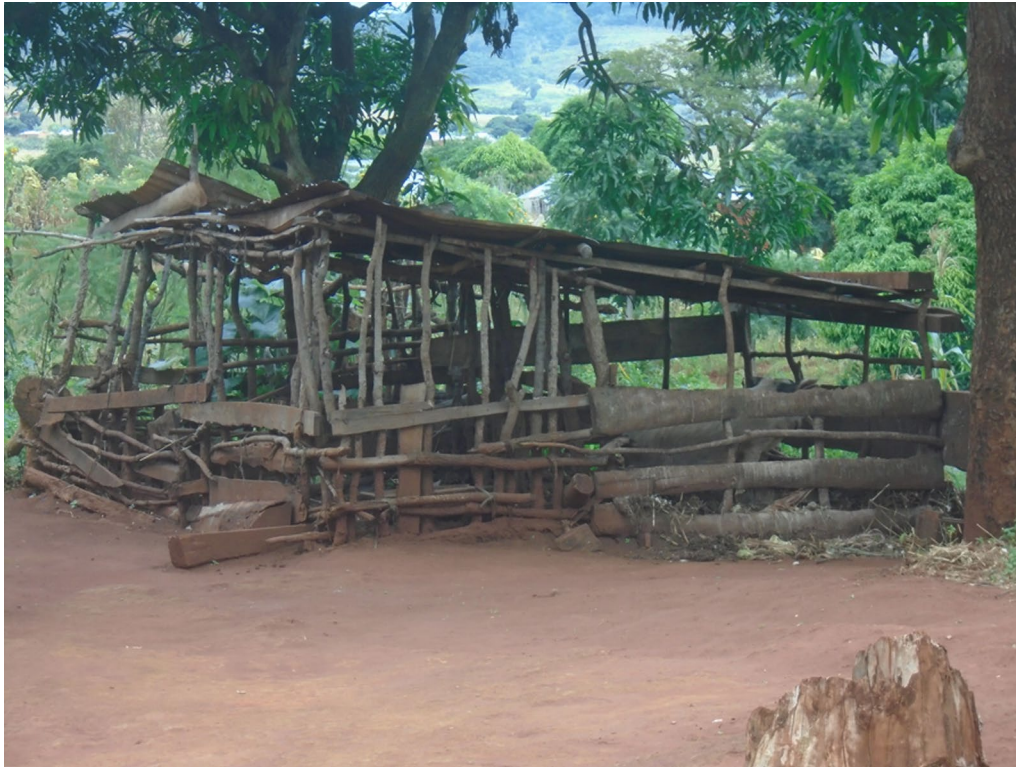
Fig. 2 Pigpen construction with clay floor and wood fence
