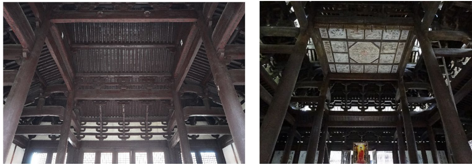
a The main hall of the Tianning Temple
