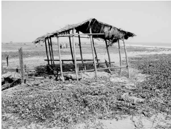
Fig. 6. Damaged hut in Kapyet Thuang Village.
