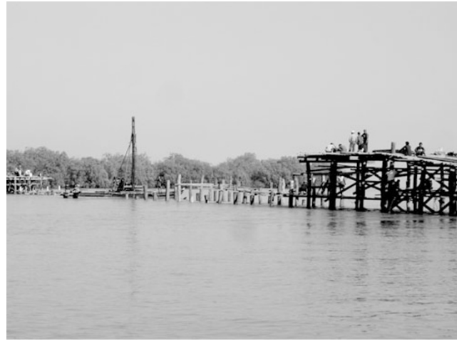
Fig. 7. Destruction of wooden bridge to Plautonton Island.
