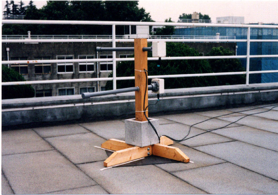
Fig. 1. Illustrating the antenna system on the roof of one of the buildings on Shonan Campus. Each antenna unit consists of a ferrite-coil antenna and a pre-amplifier. The two axes are oriented in the north-south and east-west directions.
