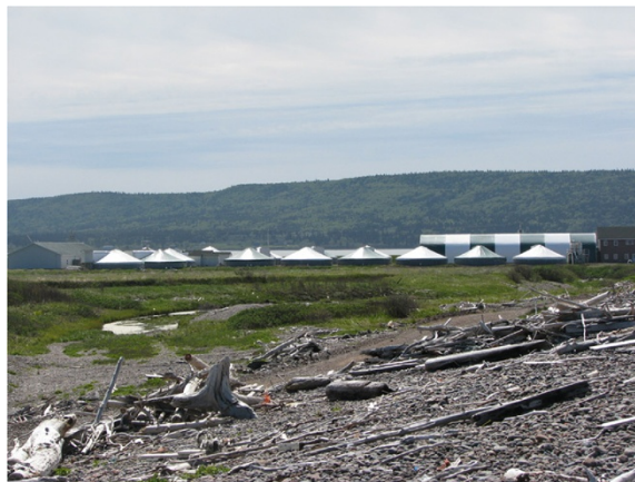
Figure 1 West Advocate Harbor NS. Looking at a north side view.
