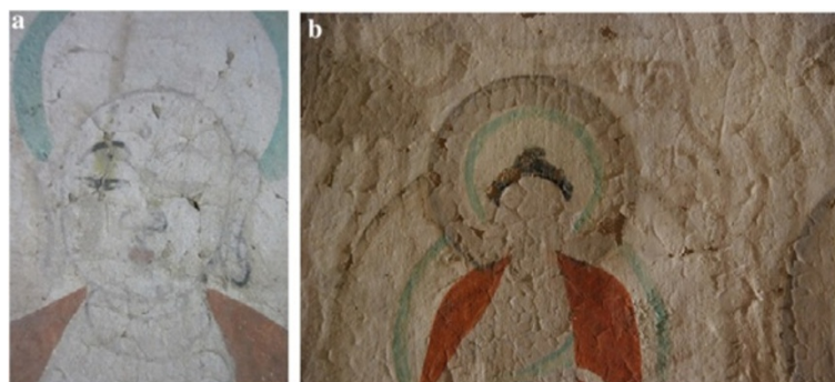
Figure 5 Pictures of flaking. (a) flaking on the center column in the 44th cave. (b) flaking after using gelatin solution to repair.
