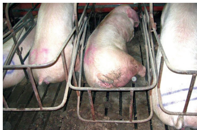
Figure 2: Build-up of faeces behind the sow and damaged stalls in the dry sow house.
