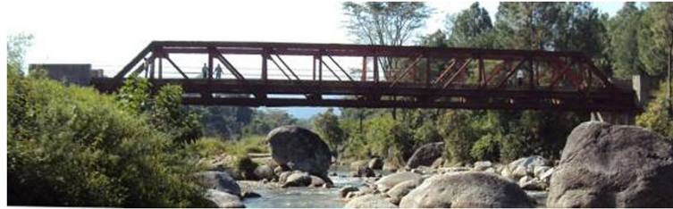
Figure 1 Side view of 40-m steel truss bridge.
