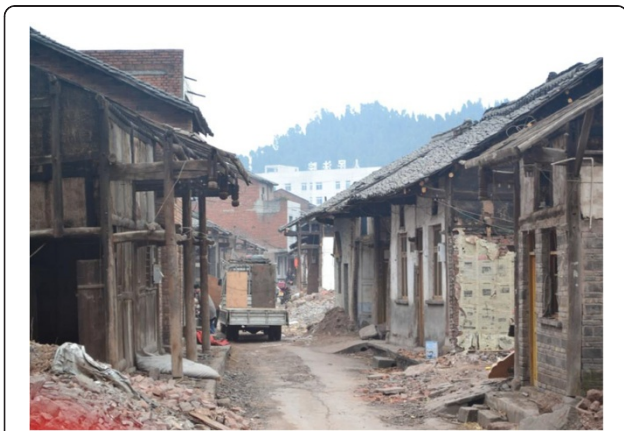
Figure 1 Collapsed houses in Guangyuan after the earthquake.
