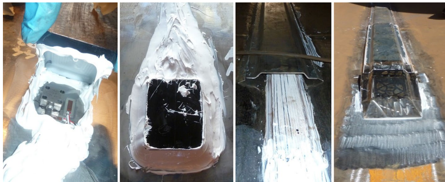
Fig. 9 Sensors below encapsulation, encapsulated sensors, cables embedded in adhesive and cable protection duct, driving shoe at end of cable protection duct near pile toe ( from left to right )
