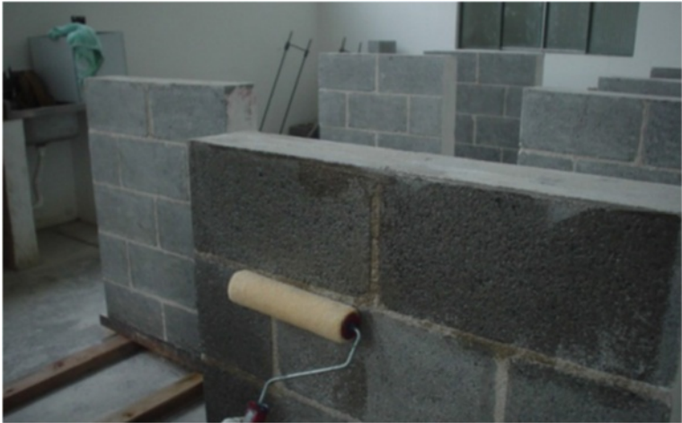
Figure 3 Application of the primer on the damaged wallets.
