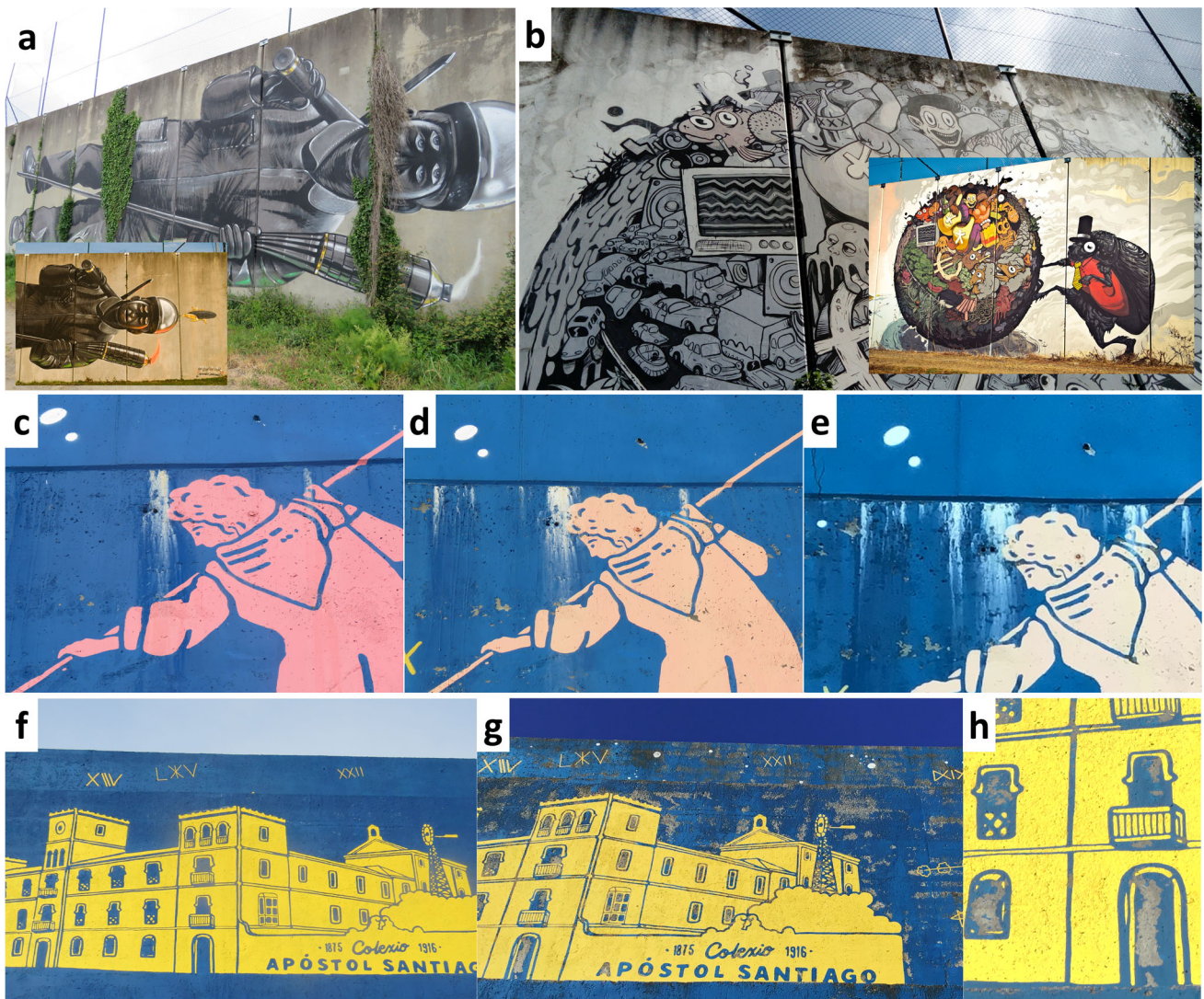
Fig. 2 Fading affecting AW20 (a), AW18 (b) and AW21 (c–h) artworks; c–e images of a detail of a pink-painted iconography from AW21 taken in 2018 (c), 2019 (d) and 2020 (e); d–f images of a detail of a yellow-painted iconography over the blue base paint of AW21, showing the progression of the deterioration from 2018 (f) to 2020 (g and h)
