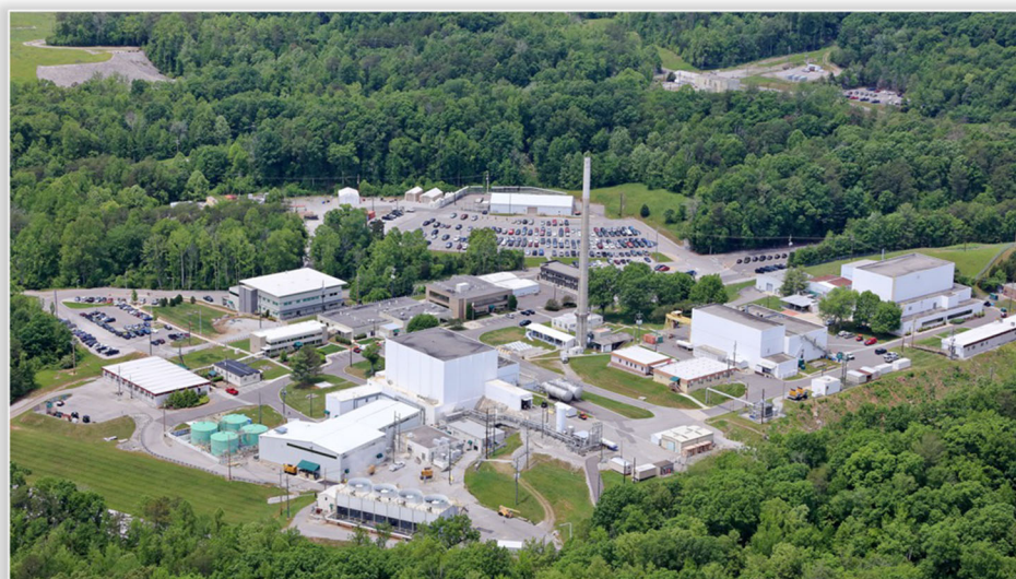
Fig. 12 ORNL's research reactor and radiochemical processing complex (HFIR/REDC)
