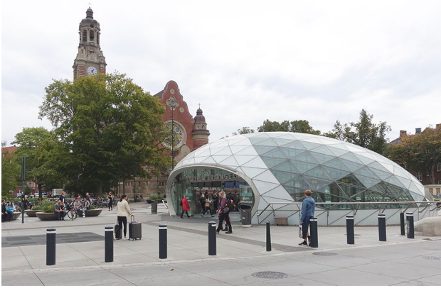
Fig. 2 Triangeln, Möllevången: a new public space dating from 2010 in the centrally located dense working class district of Möllevången (Matthew Carmona)
