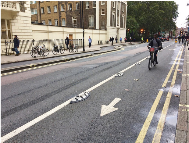
Fig. 7 Exploratory cycleway layouts (to the right of the image) in London's Bloomsbury, implemented at minimal cost prior to more permanent investments (to the left of the image) being made (Matthew Carmona)
