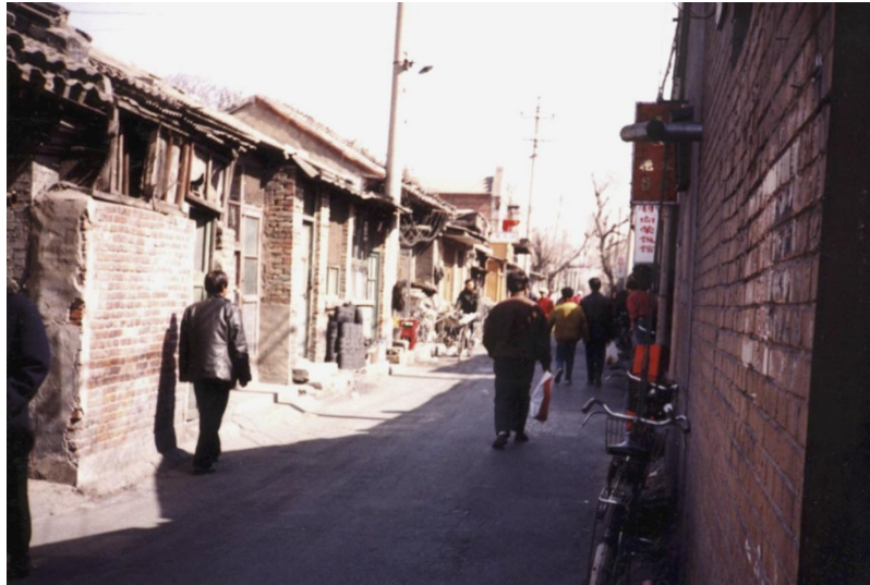
Figure 17. Deteriorated hutong ('lane') in Beijing. Note: In 1949, Beijing had over 7000 hutong. In the 1980s, the number of hutong reduced to about 3900. Today, there are only a little more than 1500 hutong left in Beijing, as Zheng (2005) noted.
