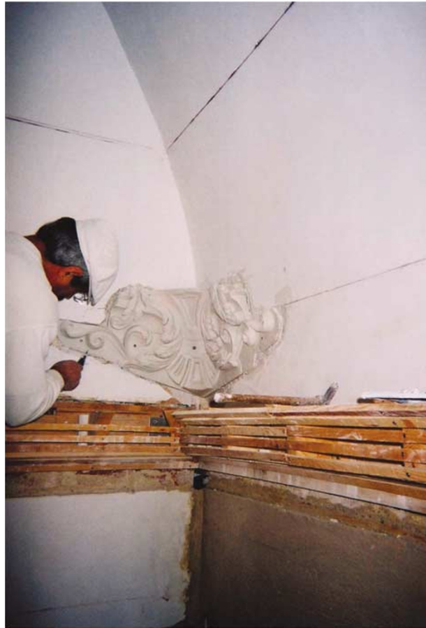
Figure 1: Reinstatement of the decoration in gaps of great dimension in a ceiling (Freixo Palace in Porto) (Cotrim et al. , 2006)
