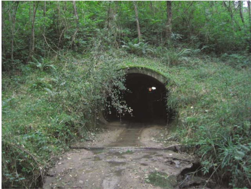
Figure 1: SW entrance of the duct ( x=0 m)
