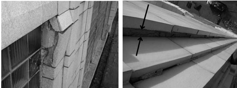
Figure 10: Examples of displaced individual terra-cotta units (left) and entire wall area (right)
