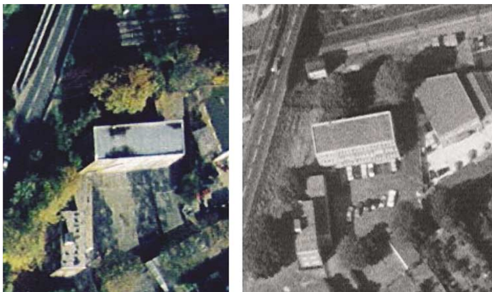
Figure 7: 1995: rainwater outlets blocked (left) and 1970: cars parked against south wall (right)
