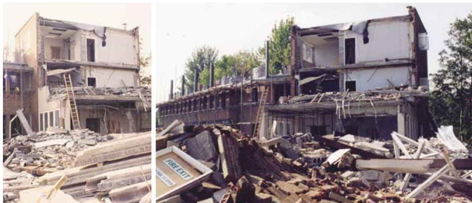
Figure 4: The building after the recovery of the bodies
