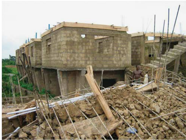
Figure 5: Clearing debris on the collapsed hotel building site.
