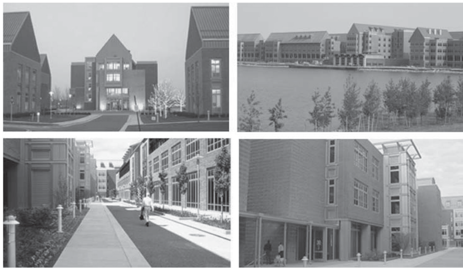
Figure 7: Visteon village ( http://www.walbridge.com/index.cfm/Projects ). Owner: Visteon Corporation; Location: Van Buren Township, MI; Market: Office; Service: Construction Management; Size: 870 000 square feet; Region: Midwest; Design Partner: Smith Group; Awards: Sustainability Design Award – American Institute of Architects 2006 Honor Award – American Institute of Architects Construction and Design Award – ASHRAE Detroit Chapter 2006 Construction and Design Excellence Award – ESD.
