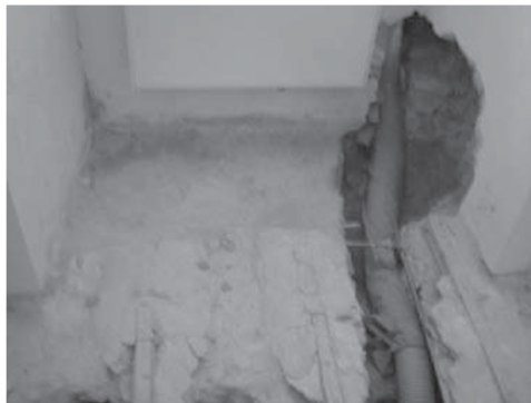
Figure 16: Introduction of the ventilation tube in the underground tunnels.
