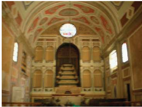
Figure 2: Church with lime plaster simulating marble.
