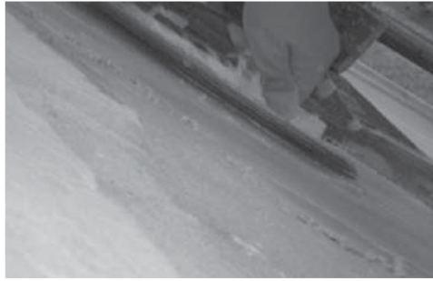
Figure 17: Application of the lime finishing coat.
