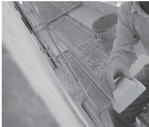
Figure 18: Finishing with the passage of a polystyrene sponge on the mortar.
