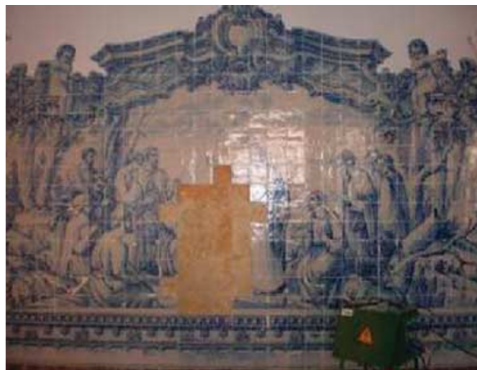
Figure 3: Lacuna in the interior glazed tiles ('azulejos') showing the old lime plaster.
