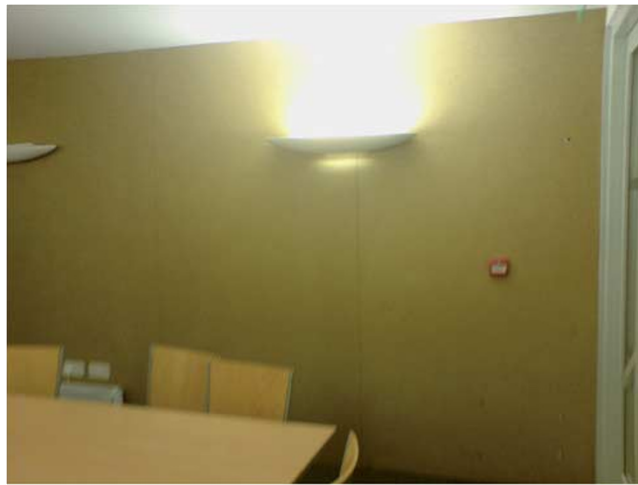
Figure 5: The flax board partition in Seminar room 1, gaps are visible between the boards.
