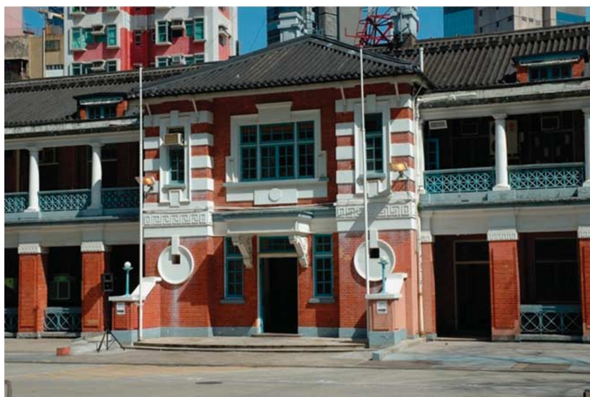
Figure 1: Front elevation of the Victoria Prison
