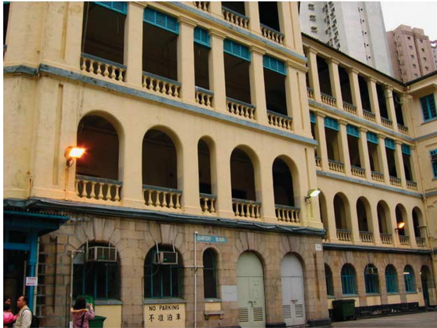
Figure 2: Rear elevation of the Central Police Station
