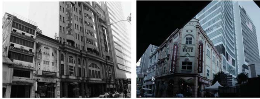
Figure 16: The pictures illustrate the contrast between architectural styles of different buildings in Tun Perak Street. Note: In most parts of the street, old ruined buildings are seen beside high rise buildings and only few historical buildings have been conserved. So there is no harmony and integrity between different buildings at the street.
