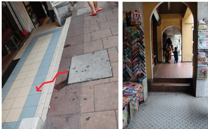
Figure 17: The steps on the pavements without ramp in Bukit Bintang Street (left picture) and Tun Perak Street (right picture). Note: These steps are a kind of barrier for people with wheelchair or pram. So the studied street have inadequate facilities for disabled people.
