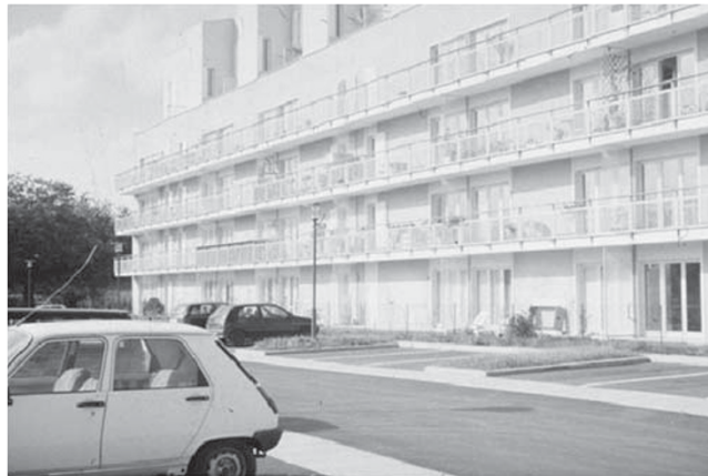
Figure 4: Salvatierra apartment block in Rennes, France.
