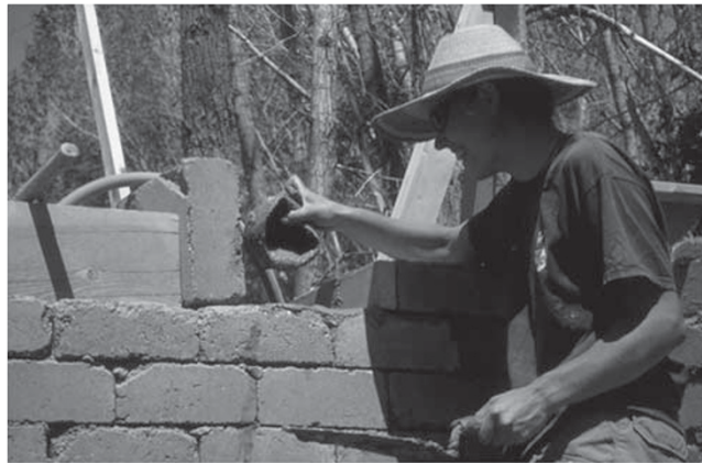
Figure 5: Laying compressed earth blocks with slurry mortar in Southern Colorado.
