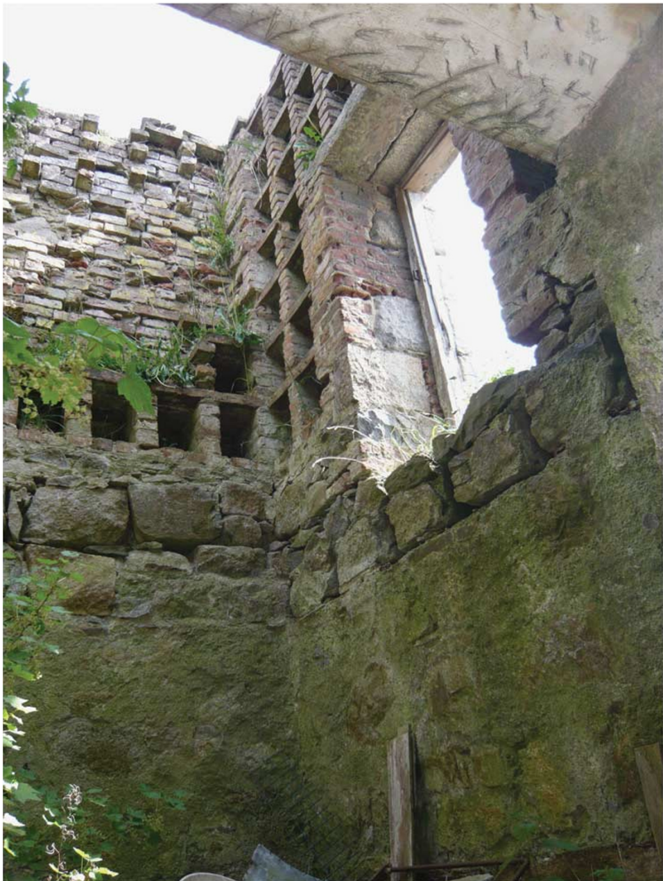
Figure 5: Interior of Blairs Doocot: Note how the projecting bricks at upper level provide a series of perches for adult birds.
