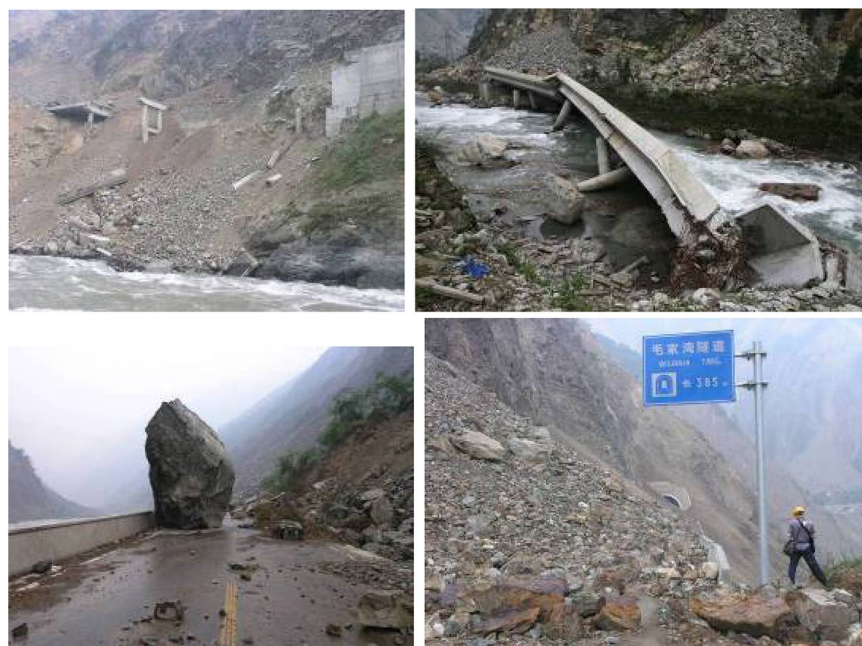
Figure 3. Slope rock mass landslide in 5.12 Wenchuan earthquake destroys a bridge, blocks the road, buries smashes tunnel entrance.
