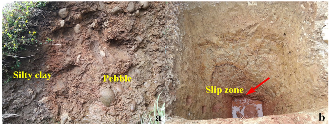
Figure 7. The structure of the sliding mass and the slip zone of the landslide exposed by exploratory trench.
