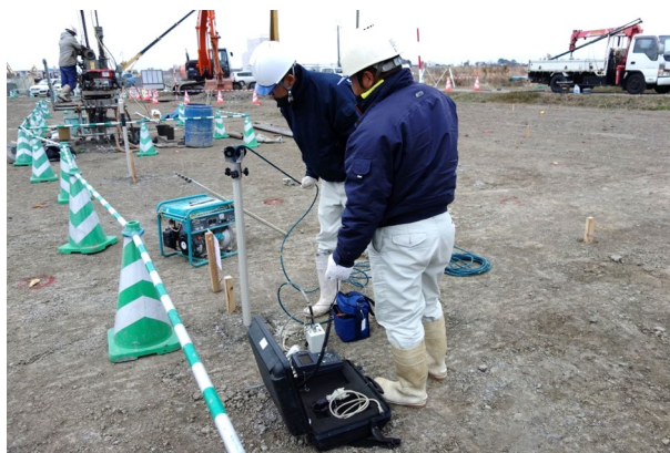
Fig. 8 Ground displacement measurement using inclinometer
