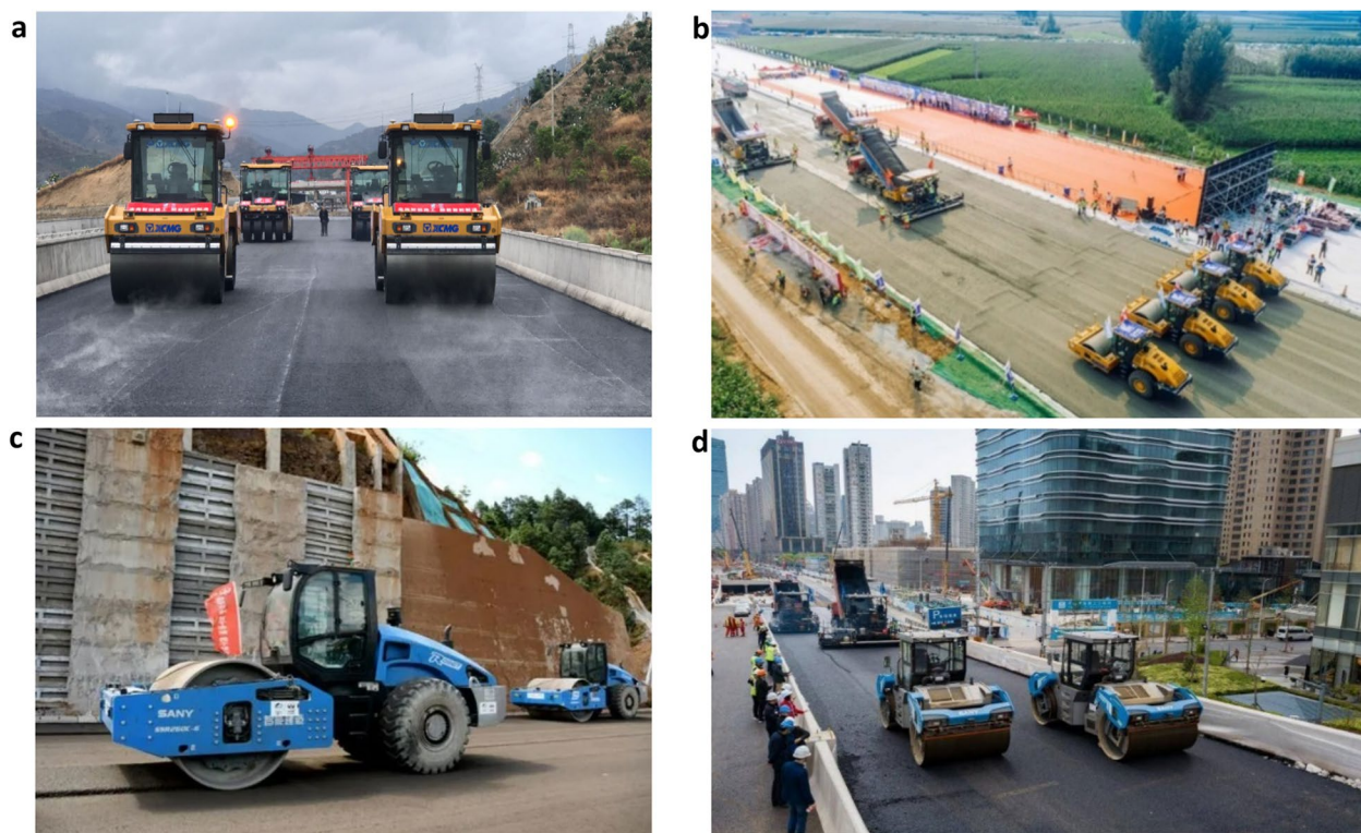
Fig. 8 On-site Construction scene for unmanned roller fleets [122–124]. a Panzhuhua-Dali Expressway. b Beijing-Xiongan Expressway. c Yangliu-Xuanwei Expressway. d The Viaduct in Shanghai
