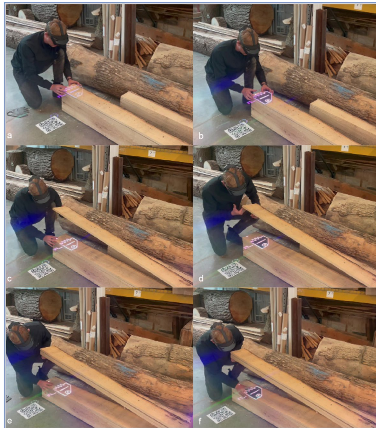
Fig. 11 Object identification is utilized to identify physical components and display intuitive step-by-step assembly instructions
