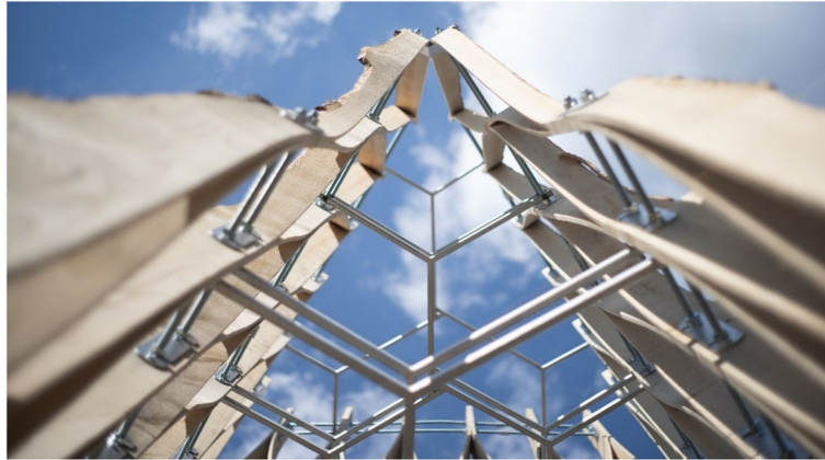
Fig. 13 Reciprocally framed tube steel in the UnLog Tower , photo by Cynthia Kuo.
