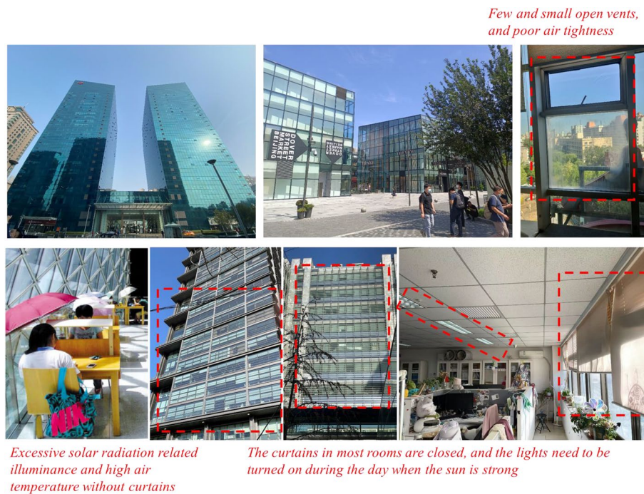
Fig. 11 Some of the problems found in glass curtain wall buildings
