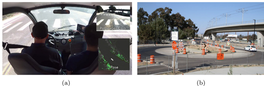
Fig. 23 An intersection (a) was converted into a round-about (b)
