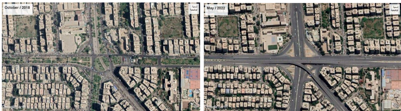
Fig. 1 Al-Hegaz Square before and after renovation. Both maps were exported from “Google Earth Pro”. The image on the left was exported in October 2018 and the one on the right in May 2022. No editing applied, and the difference between the colors of both satellite images is due to the conditions of each photo in Google Earth
