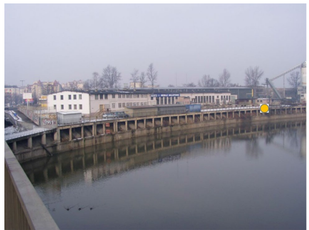
Fig. 6 General view of the considered RC river wharf
