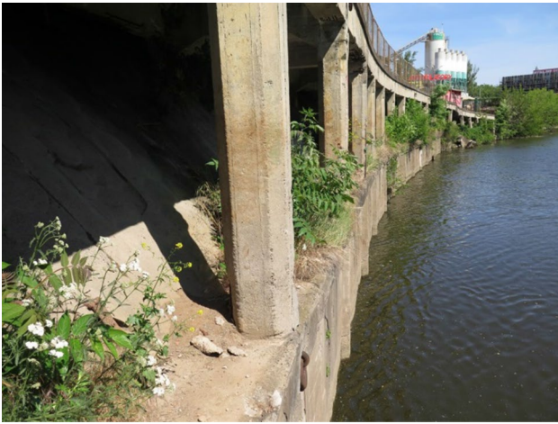
Fig. 7 View of part of the RC river wharf
