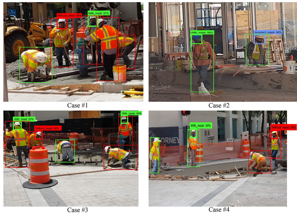
Fig. 5 The application of the model on four road construction cases
