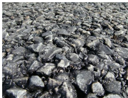
Fig. 2. Macro- and micro-texture of PAC mixes after approximately 8 years of service.
