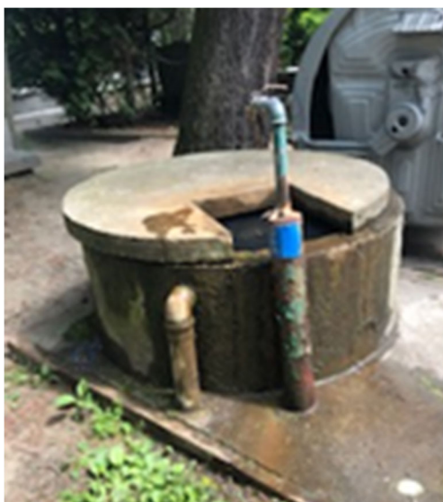
Fig. 2 An example of a water supply well widely present in selected Wrocław cemeteries
