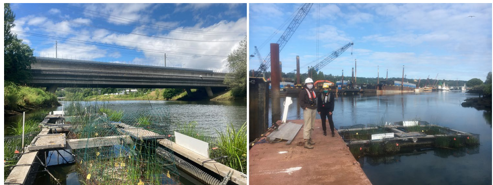
Fig. 2 Images from June 2022 (left) and April 2022 (right) showing the floating wetland “Biobarges” (the larger monitoring structure) with floating wetland “Biofilters” and monitoring equipment attached, deployed on different sections of the Duwamish River Estuary, and pictured with Community Scientists. [Image credit: the Duwamish Floating Wetlands Project Team, UW Green Futures Lab]
