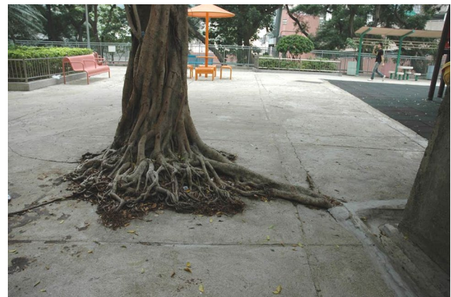
Fig. 3 This Ficus microcarpa (Chinese banyan) planting site is sealed by recently laid pour concrete up to the trunk base, even though the recreational open space has low pedestrian traffic (Homantin Estate, Kowloon, C. Y. Jim photograph)
