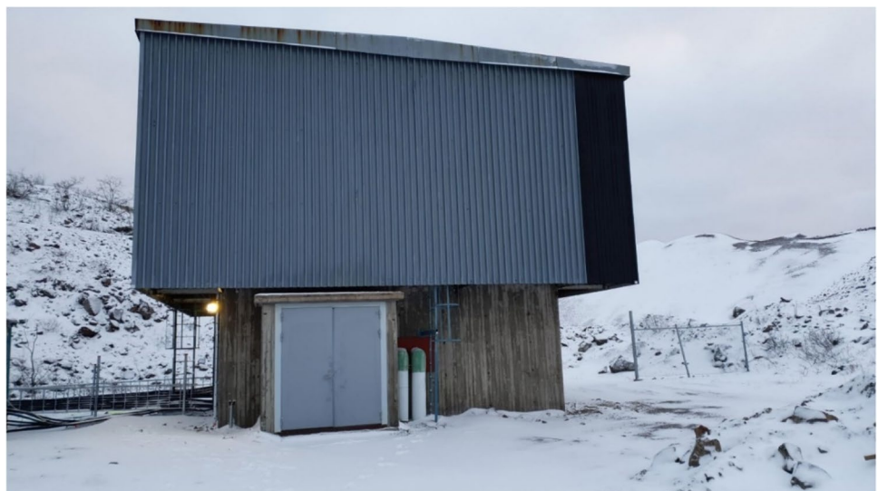
Fig. 5 The building housing Konsuln's direct contact electric heating system
