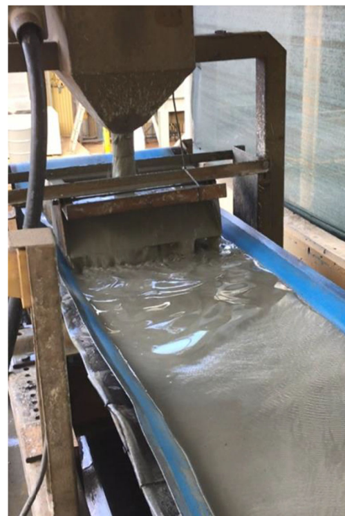
Fig. 3 Filter feedbox and overflowing weir distribution system
