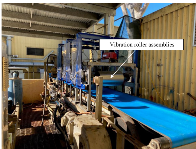
Fig. 2 Pilot vibration roller assemblies
