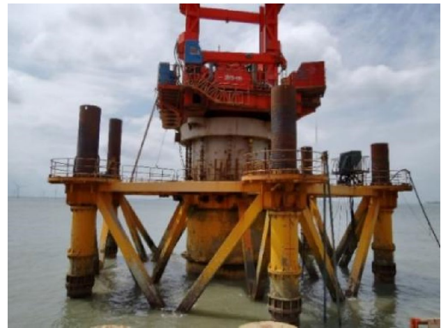
Fig. 1 The large diameter offshore drilling platform
