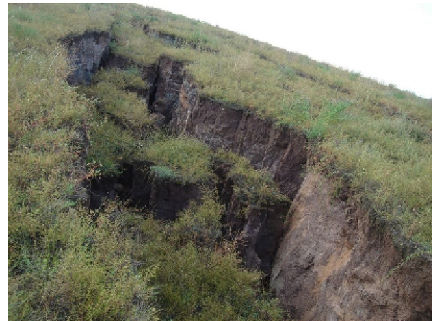
Fig. 6 Discontinuous surface cracking of the 12,401 ground subsidence basin
